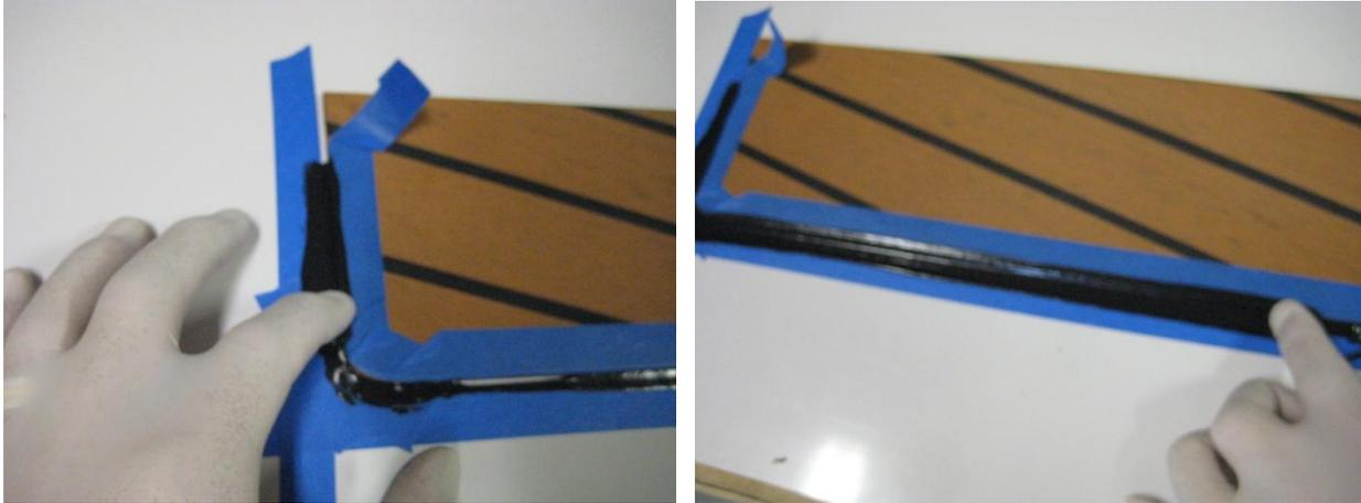
You want to really press firmly and make a perfect fillet from the edge of one piece of tape to the edge of the other. If the caulk is too thick it will cause problems when you remove the tape.
